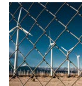
Power Generation Security
